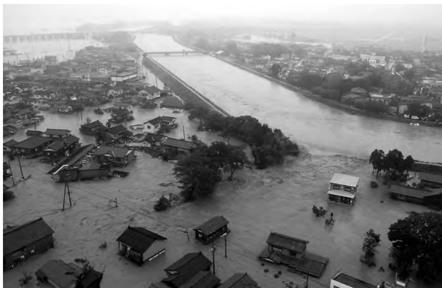
Photo 2. Flood water flowing into the housing area from the bank break site of Kariyata River (Photo by Kyodo-Tushinsha).
